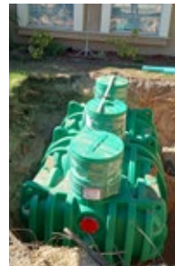
Installation of an advanced-treatment septic system
